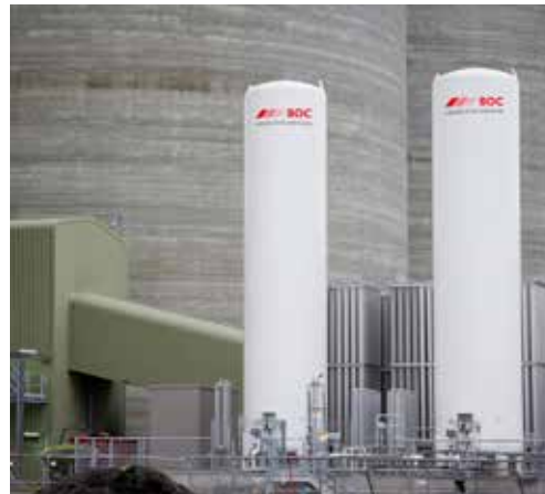
BOC Biomass Fire Suppression system
